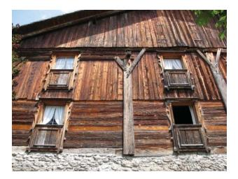
Figure 1. Post-and-beam construction, Sulz
